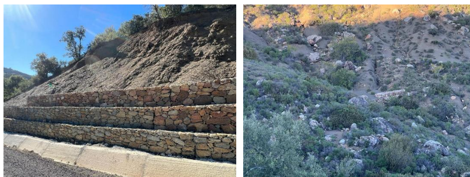
Figure 6. Types of management practices in the watershed (threshold gabions in streams and along roadbanks).
